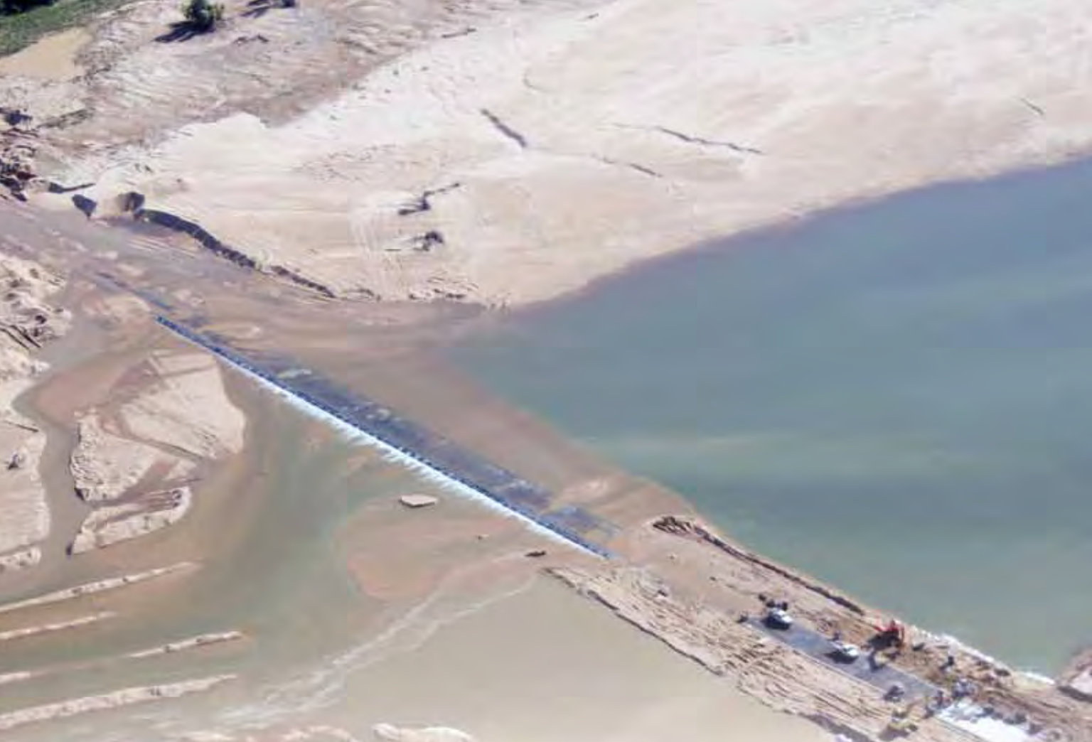
The crossing during installation of its total 400 metre length.
