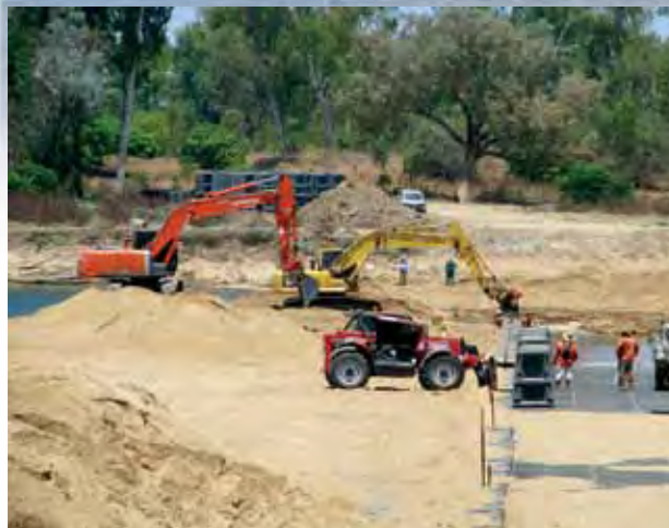
Building a sand island to form the crossing.
