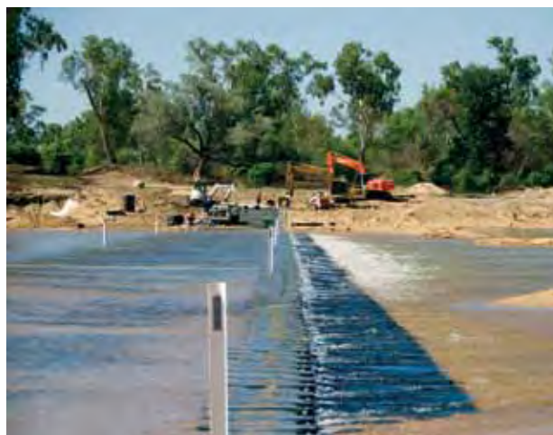
Water flowing over the completed crossing.
