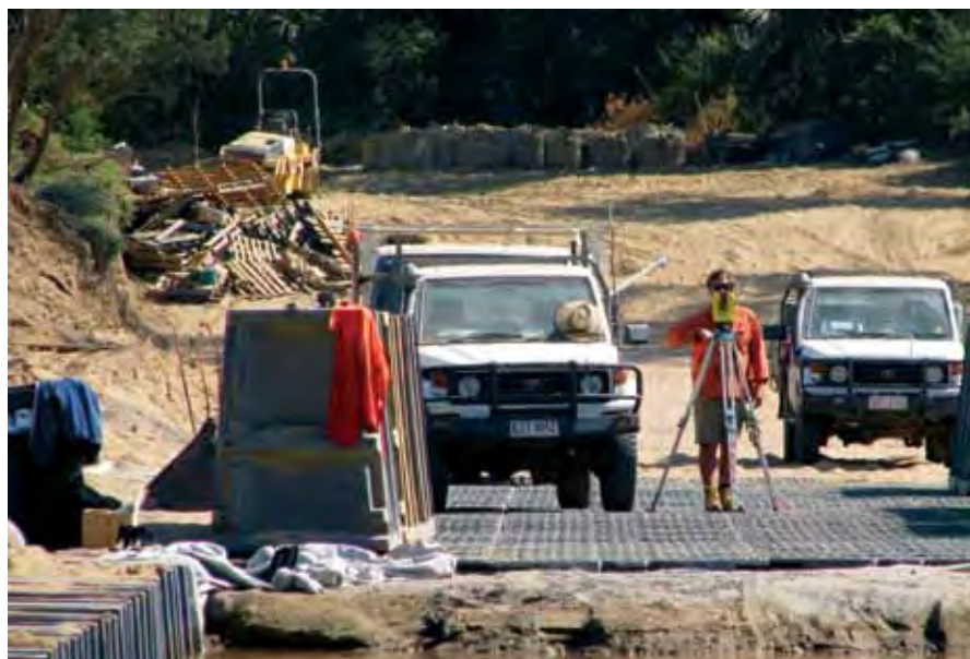
Checking levels on the crossing prior to installation of the system.
