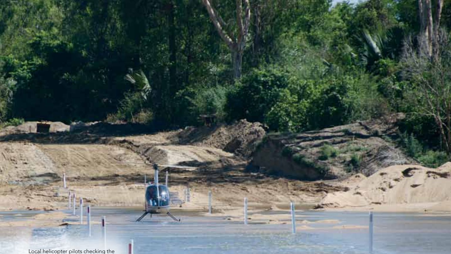
Local helicopter pilots checking the progress of the new crossing.
