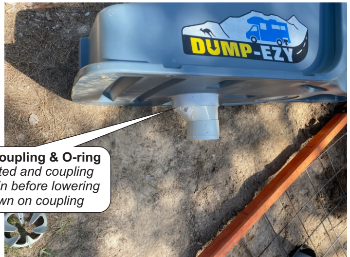
100mm Fernco Push Fit Coupling Allows unit to be unbolted and easily lifted up if access to the plumbing is ever required for maintenance. eg. a blockage If PVC L.I.T is solvent glued you cannot remove the unit without breaking the plumbing.
