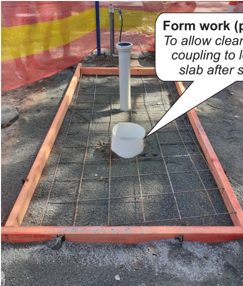
100mm Fernco Push Fit Coupling Allows unit to be unbolted and easily lifted up if access to the plumbing is ever required for maintenance. eg. a blockage If PVC L.I.T is solvent glued you cannot remove the unit without breaking the plumbing.
